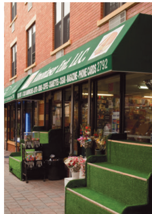
Community developments like Cypress Plaza Mews, Brooklyn are needed to revitalize low-income neighborhoods. Photograph: courtesy Local Initiatives Support Corporation
